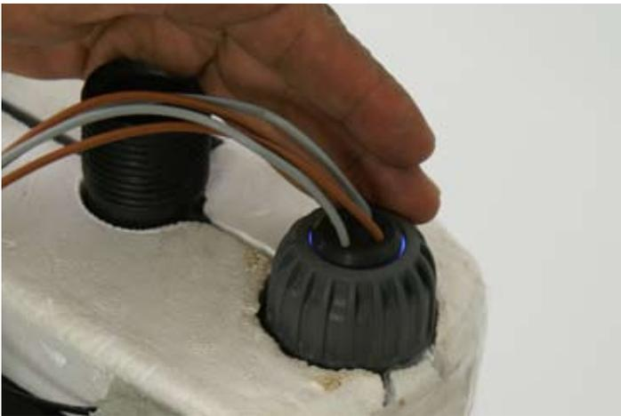
You should see a glow around the rim of the quartz sleeve indicating the UV is working. Immediately turn off chiller after verifying the lamp is working.
