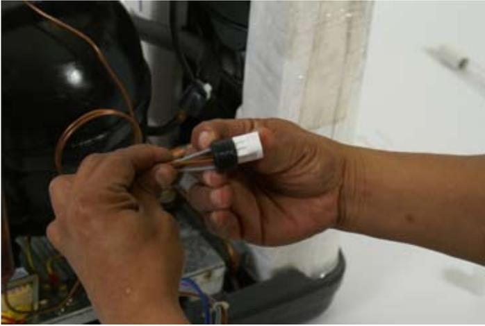
Slide the rubber plug along the wiring until it is directly against the 4-pin connector.
